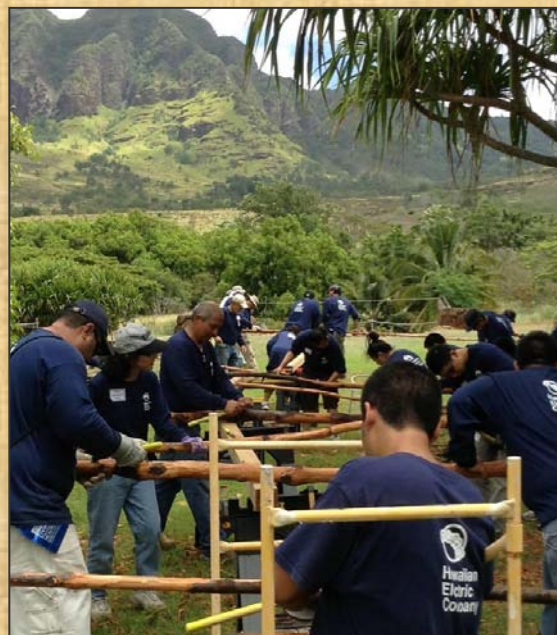
Rebuilding Hale Na'auao in July 2013
